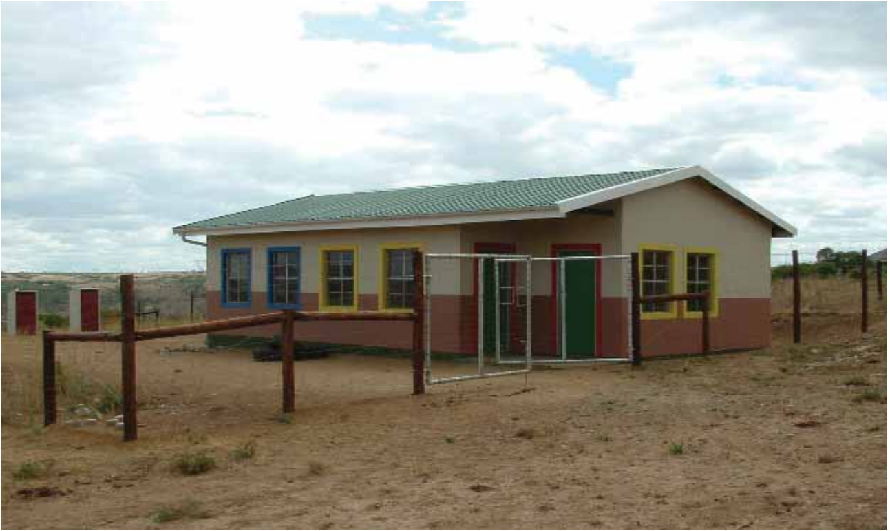
Zulu Rock Creche with VIP & fencing
