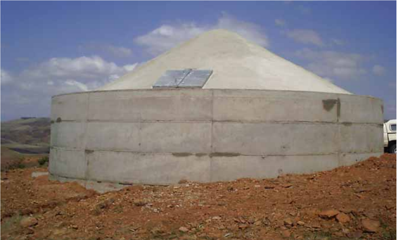
Reservoir constructed at Simdlangetsha west regional scheme
